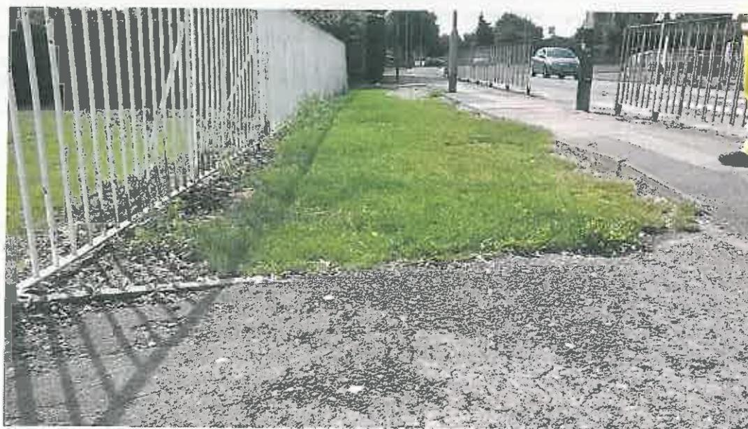
**Photo No. 2. - View North End of Verge Showing missing and Uneven Edge Stones**
