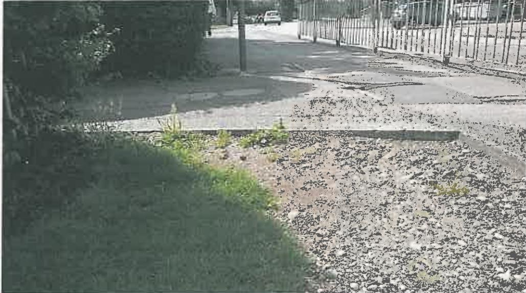
**Photo No. 3. - View of South End of Verge Showing Degree of Settlement Within Verge.**
